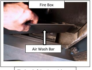
The bend of the air wash bar should face TOWARD the front door
